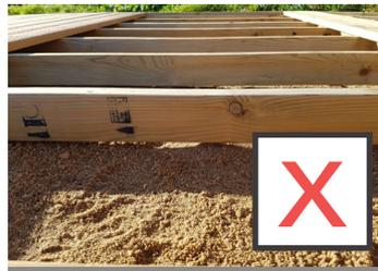
Base substrate not a solid material making the base unable to support heavy structures.
