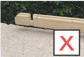
Concrete base running out of level by more than 10mm.
