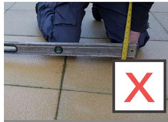
Slab base has a water run-off allowance making the base run out of level by more than 10mm.
