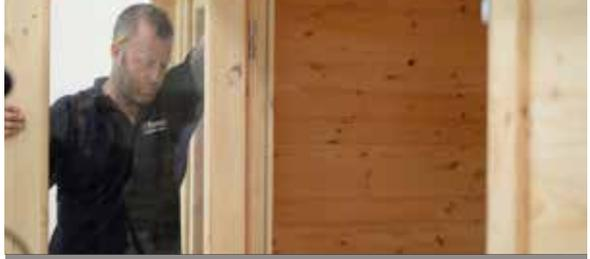
Line up the male and female parts of each hinge and lower the doors into place.
