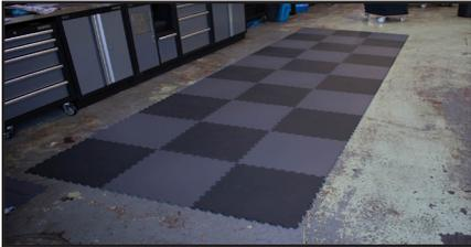
**Step 4:** Continue to add tiles forming a pyramid (Refer to the numbering system below).
