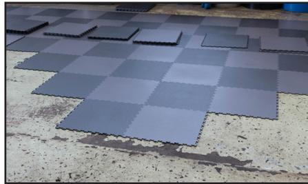
**Step 5:** Continue to build the staggered pyramid by adding one full size tile to both ends of every row.
