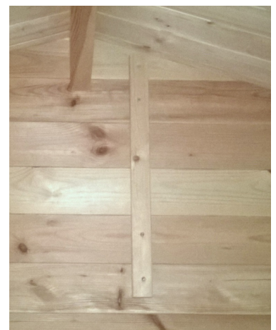
Braces can be easily installed to the interior of the cabin with an electric screwdriver.
