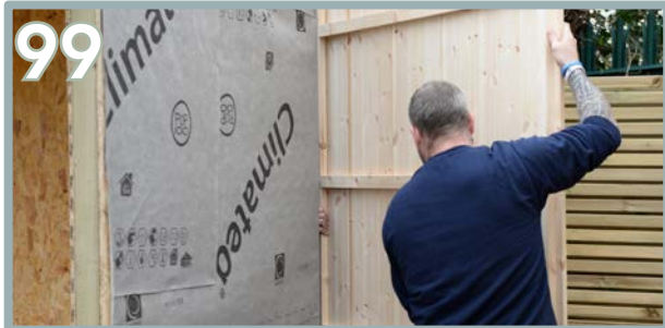
Begin applying the T&G Back Panel (AZ).
