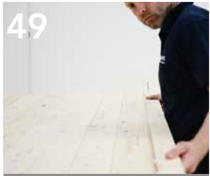
Place the cut down roof board into position. Pre-drill and screw once to each rafter.
