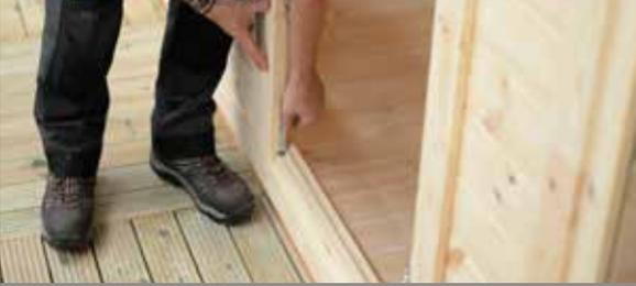
Ensure the shoot bolts located at the top and bottom of each door align with the shoot bolt holes located within the door frame.
