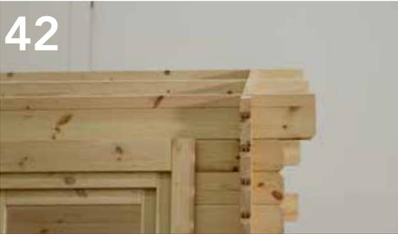
Finally insert the top rafter into the recess on each side of the cabin.
