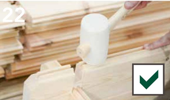
Please ensure a rubber mallet is used at all times when striking the logs. Always strike the logs on the inside of the joint.
