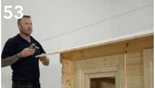
Apply a chalk line on these two measurement points and mark a line across the entire width of the cabin.
