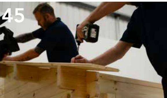
Place the edge of the first roof board flush with the edges of the rafters. Pre-drill and screw each roof board twice to each rafter working your way from one side of the cabin to the other.
