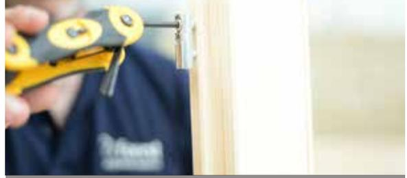
If the doors need adjusting, lift them back off the hinges and use an Allen Key to adjust each hinge accordingly.
