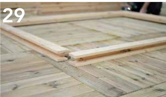
Assemble the door frame. The door frame comes with the screws pre-sited, so line all the parts of the frame up with each other and screw together.
