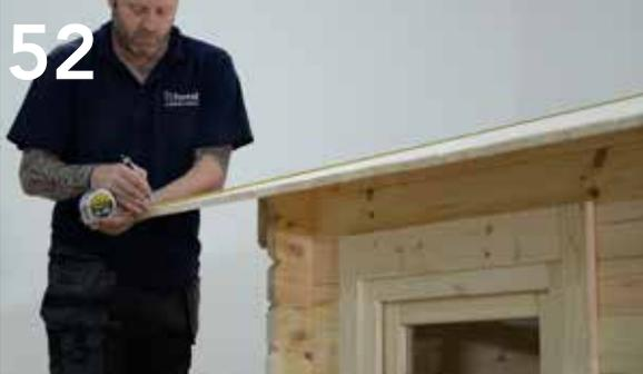
Transfer this measurement to the end board on either side of the cabin.
