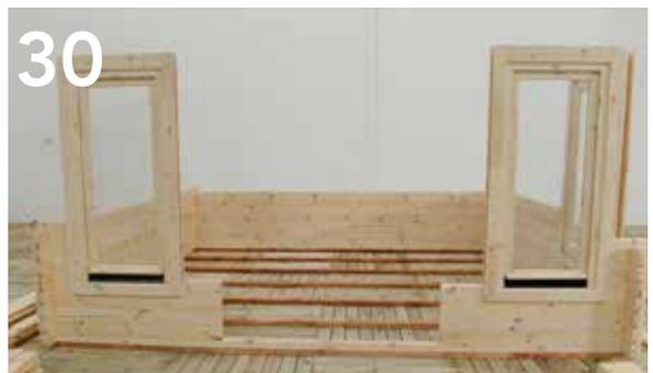
Build the cabin up to about 8 logs high then slide each window frame over the logs. This will help act as a guide for all additional logs.
