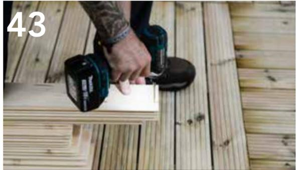
Pre-drill two holes in the top of each roof board. Do this on one end of each roof board only, this is the end that will attach to the middle rafter.
