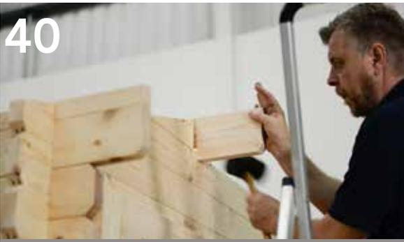
Take two of the three remaining rafters and fit each one tight against the recess on either side of each apex.
