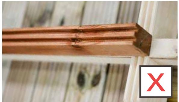
Do not lay the floor bearer on its narrowest edge otherwise the internal lip to support the floor boards won't be created.
