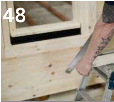
Proceed to cut the roof board down to size.
