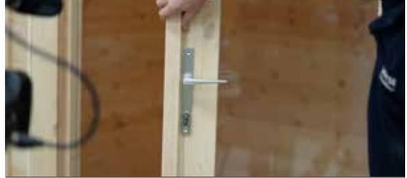
Place the handles into position and secure by tightening the small grub screw on the side of one handle.
