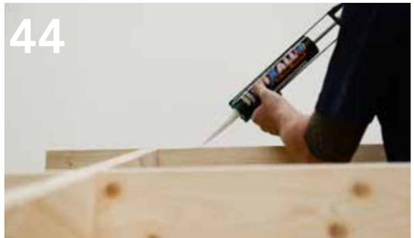
If applying adhesive, only apply enough to each rafter for three or four roof boards at a time as it's quick drying.
