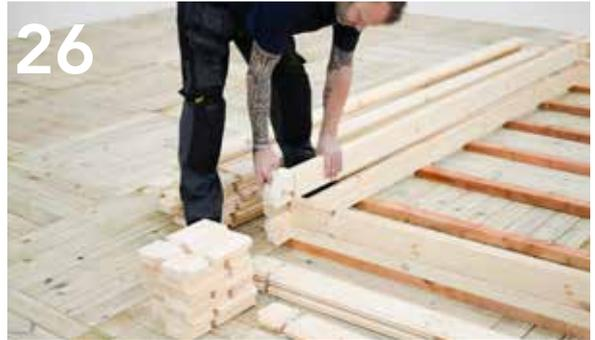
Interlock a side log over the front and back rear logs.
