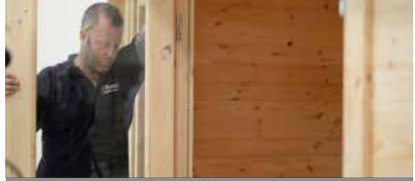
Line up the male and female parts of each hinge and lower the doors into place.
