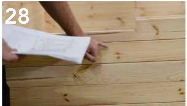
Build the logs up to window height. Referring to the instructions, note how many logs are needed to be installed before the window recess log is installed.
