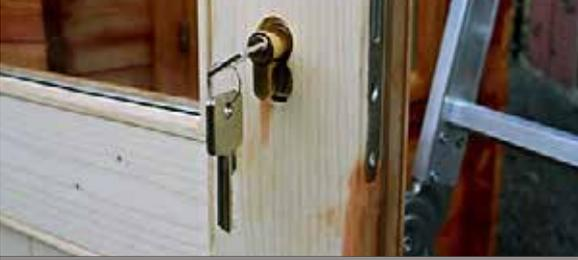
Firstly locate the Euro Cylinder into the mortice lock. Use the keys and turn slightly allowing it to fit in.
