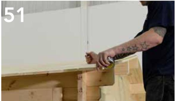
To do this, locate the shortest board and measure the distance between the apex point of the roof and the end of the board.
