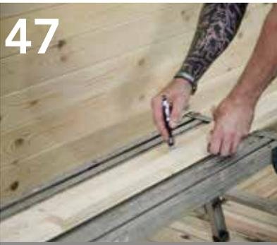
Using a straight edge join the joist marks together on the roof board by drawing a cutting line.
