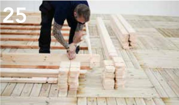
Start building the cabin walls by securing a full log to each of the half logs.
