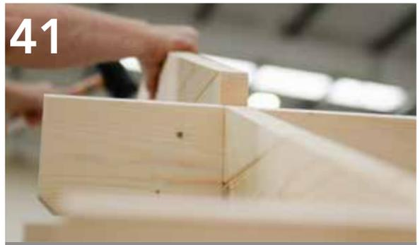
Insert the middle section of each gable end, ensuring a tight fit against the rafters.
