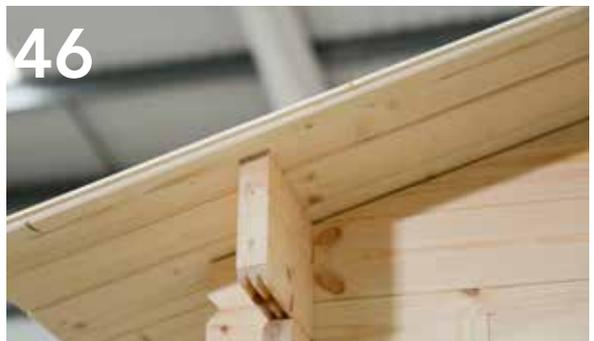
Place the last roof board into position and mark the position of each rafter edge on the underside of the board.
