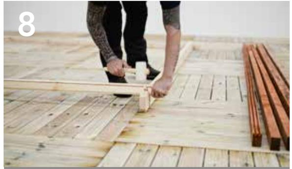
Using a white faced rubber mallet, connect the half log to the full log. Please ensure you strike the log on the inside of the joint, not on the outside where you risk snapping the end of the log off.
