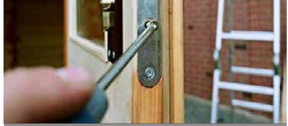
Fit the screw to secure the Euro Cylinder. If you peer through the screw hole you should be able to see the threaded hole in the Euro Cylinder, in which it has to locate. If not wiggle it around until you do.
