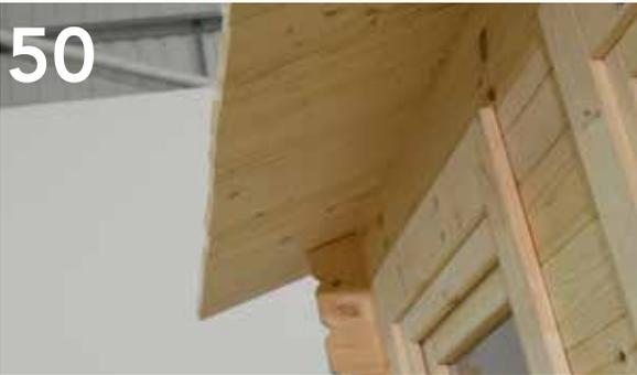
When all the roof boards have been installed the roof board edges which overhang the front and rear of the cabin will need to be trimmed flush.
