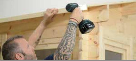
Pre-drill both ends of each strip and once in the middle (three screws per section). Before fixing into the end grain of the roof boards, ensure the top of the end grain protection strip is flush with the top of the roof boards and the end of the strip is flush with the outside edge of the end roof board.
