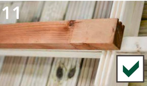
Lay the first floor bearer on top of the flat surface of the half log making sure the edges of the bearer line up flush with the outside edge of the half log. Also ensure the bearer is laid on its widest edge.
