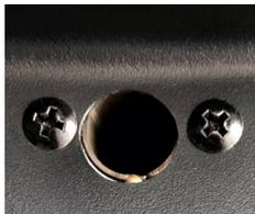
Inspection hole for visual inspection of the booster burner flame.
