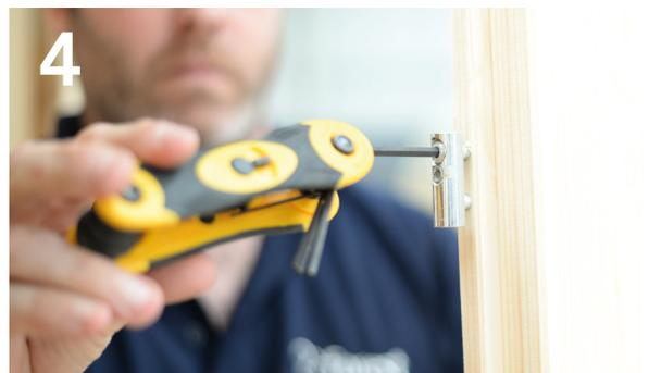
Using an Allen Key, turn the adjustment bolt anti-clockwise to push the door closer to the adjacent door, or turn it clockwise to pull the door back towards the door frame. Repeat with the bottom hinge as necessary.
